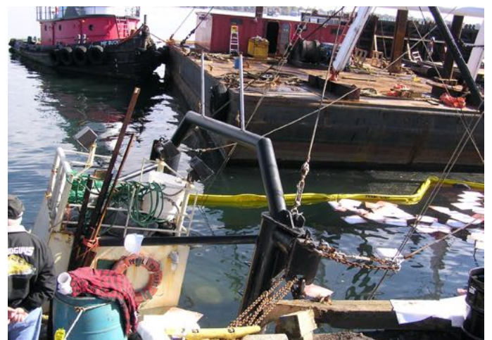
An absorbent boom and fuel pads placed in water to collect oil released from a sunken boat. Photo credit: Massachusetts DEP.
